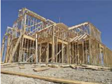
Figure 5. Lightweight timber construction;
