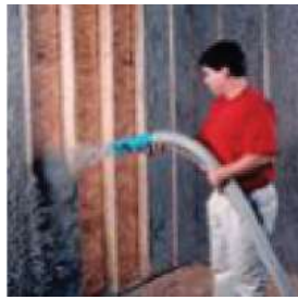
Figure 7. Spray-in-place cellulose
