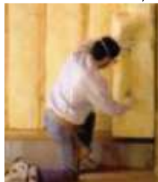
Figure 8. Fiberglass installation
